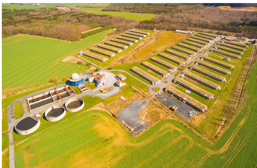
Fot. 1. Biogazownia rolnicza przy chlewni w Czechach. Fot. Kletr (oryginalny opis fotografii: Aerial view to biogas plant from pig farm in green fields. Renewable energy from biomass. Modern agriculture in Czech Republic and European Union, [[:]] https://www.fotolia.com/id/106610777 )
