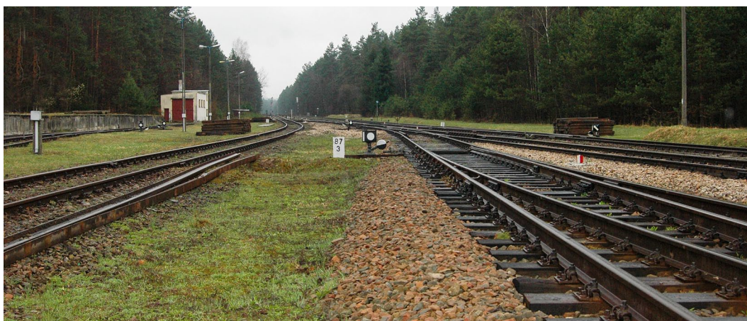
Fig. 2. Railway tracks crossing the Park. Photo by Łukasz Sędlak
