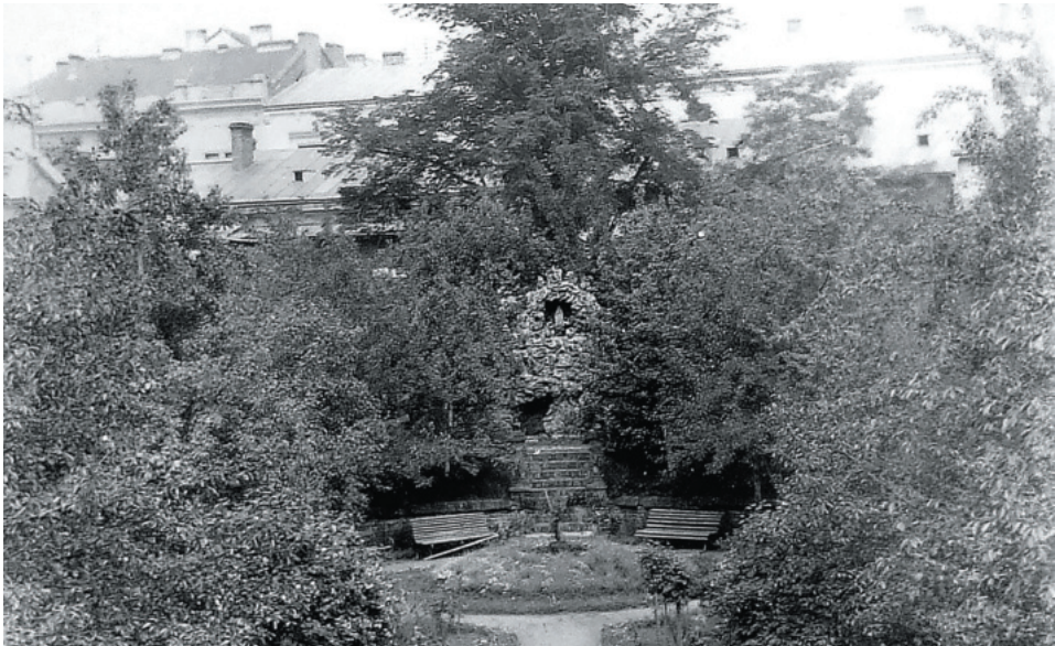
Fig. 2. Garden at the Cracow Resurrectionist house on Łobzowska Street, with the grotto of Our Lady of Lourdes. State before 1923.
